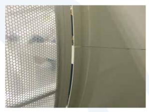
Rigid seal stops are pre-installed flush with the outside of the plenum cage before shipping. They must be adjusted before installing seals.
