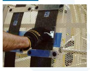
Apply pressure to seal reinforcement with supplied press tool for 1 minute.
