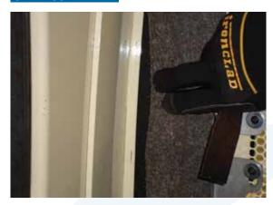
Pull back the outer edge of the secondary seal from the plenum wall and verify the correct position of the primary seal elastic retainer.
