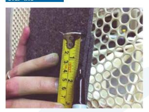
Add an additional 1 1/2" [38 mm] to overlap mark to account for primary seal thickness. Make new mark.
