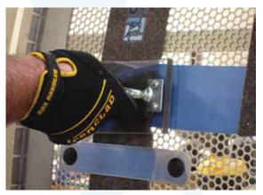
Apply pressure to seal reinforcement with supplied press tool for 1 minute and then let hot glue cure for an additional 15 minutes.
