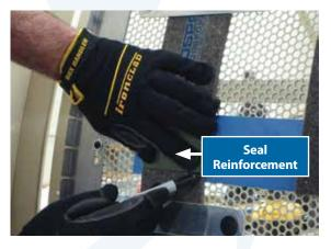
After hot glue has fully cured, center seal reinforcement over seal joint and mark the perimeter of the seal reinforcement.
