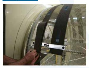
Mark the location of overlap. NOTE: Primary and secondary seals are delivered longer than needed and must be cut to length during installation.
