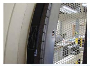
Align leading edge (closest to plenum wall) of elastic retainer on leading edge of primary seal.
