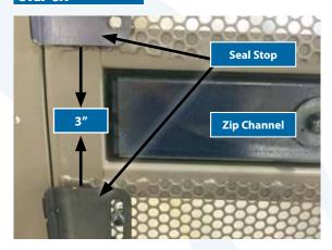
Begin installing the flexible seal stops by placing (2) of them adjacent to the zip channel which must not be covered. This will leave a gap of approximately 3".
