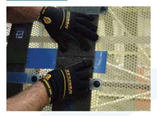
Quickly align secondary seal ends and hold together for 1 minute to allow hot glue to dry. Allow an additional 15 minutes of curing time before moving to next step
