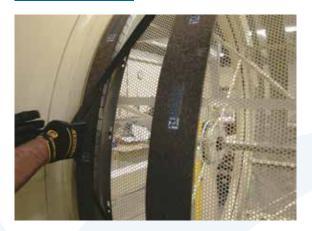
Work elastic seal retainer over seal stops towards plenum wall.
