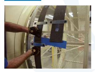
Quickly align primary seal ends and hold together for 1 minute to allow hot glue to dry. Allow an additional 15 minutes of curing time before moving to next step.
