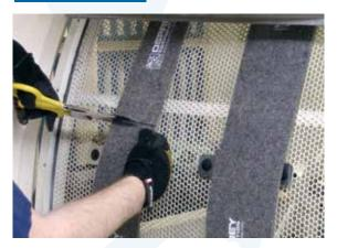
Using the supplied shears, cut seal at overlap mark ensuring that the cut is perpendicular to the sides of the seal.
