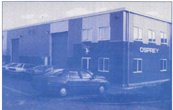
Osprey's New Facility at Whitstable
