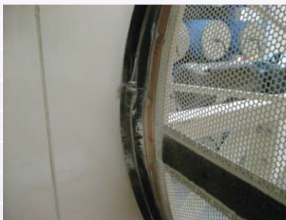
Figure 2 - Drum Seals Installed
